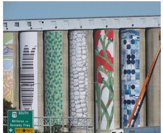
As seen along interstate 80
